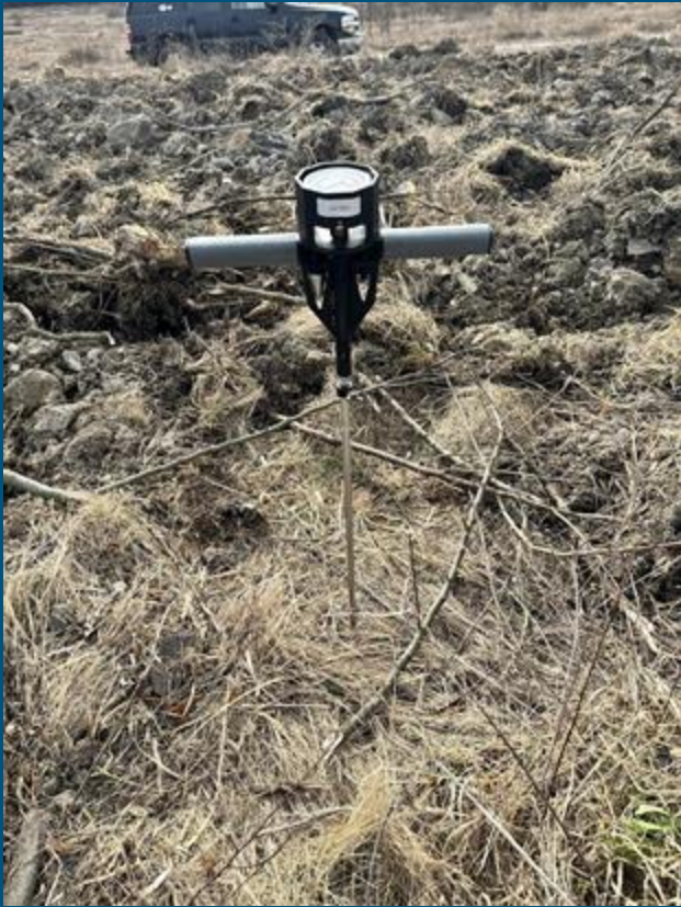
Un-ripped area- compaction
