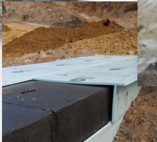
Portal extension and lime amendment
