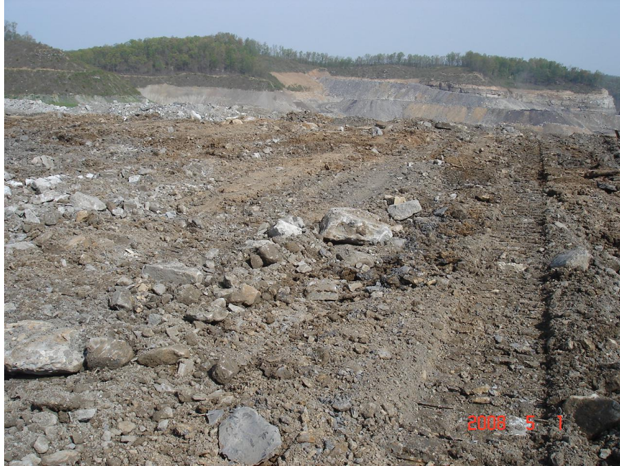
Figure 1. The 1-ha experimental area was constructed with primarily brown sandstone substrate, end-dumped with trucks, and the piles were flattened by one or two passes of a bulldozer.
