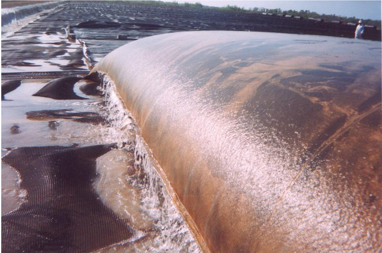
Figure 4. Typical Geotube® Container Installation
