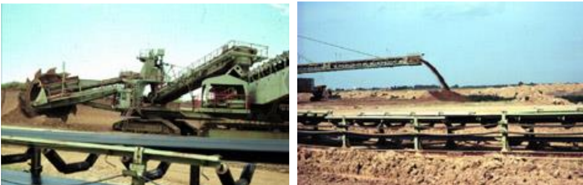
Figure 7. Captain wheel-conveyor- spreader system resulting in low strength soils
