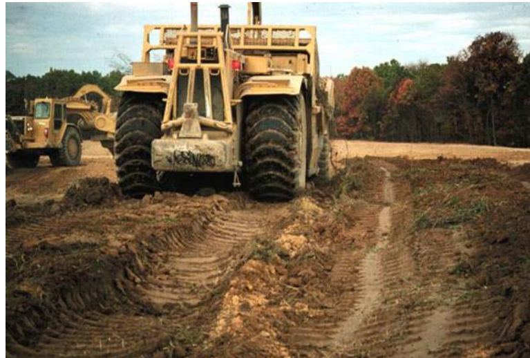
Figure 4. Scraper haul system replacing soil materials with high axle load on rubber tires results in high strength soils
