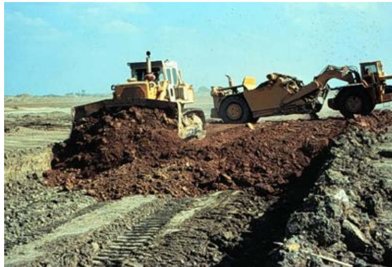
Figure 1. Placing B horizon material at Sunspot mine
