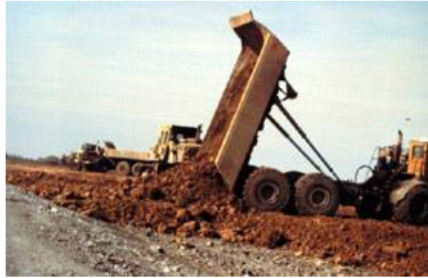
Figure 10. Rear dump trucks replacing root media with traffic on media (TWT)
