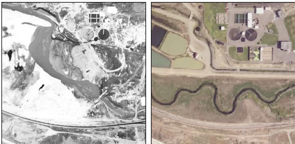
Figure 4. Aerial photographs of the Silver Bow Creek floodplain at the east end of the Colorado Tailings before (1969) and after (2002) waste removal and stream channel reconstruction. Notice the municipal waste water treatment plant in both photographs.
