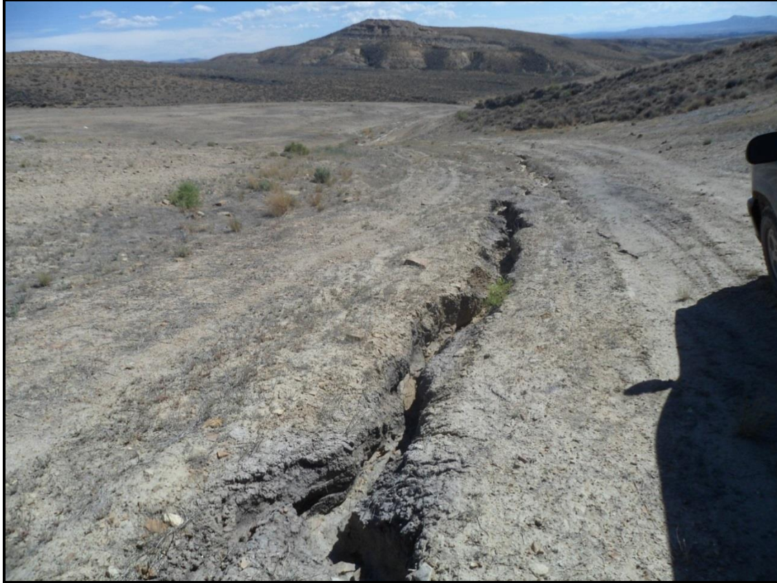
Figure 13. Traditional channel failure in the Reliance No. 11 North Pit, looking downstream. Steep channel gradient was the cause of the failure.
